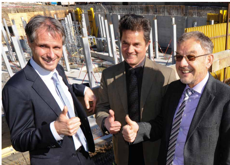
Raffaële Balmelli, Head of Implemia Ticino, Thomas Schulthess, Director of CSCS, and Roman Boutellier, Vice President Personal and Resources of ETH Zurich, during the foundation stone ceremony on the construction site.
